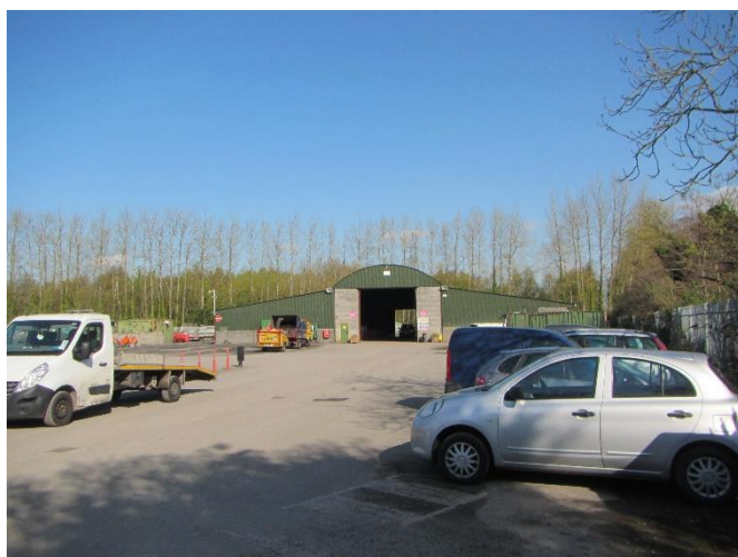
Photograph 9 The yard and corrugated sheet shed.
